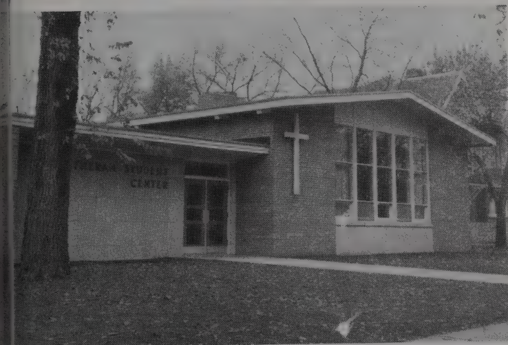
Lutheran Student Center (completed 1957)
